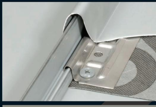
The Seam over cloak fits over the Locking Leg and snaps into place. The Locking Leg is profiled with an anti-siphon design which doubles up to eliminate capillary action in the joints and forms the 'Receiver' to which the MS secret fixing clip is placed to secure the panel to the substrate.
